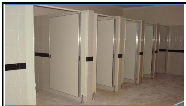
KAMAR MANDI / TOILET
